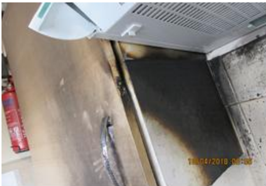
Fire damage in shared kitchen
